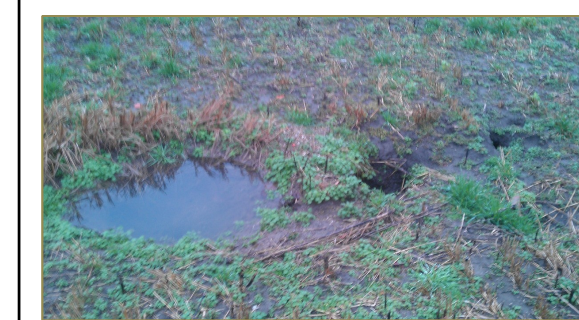
Figure 4. Tile blowhole and standing water
