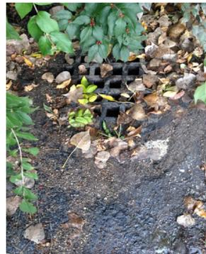
Figure 3: Current drain blocked
