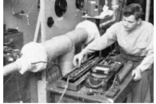
Thermosyphon loop used to determine boiling heat transfer coefficients in two-phase flow (1954).
