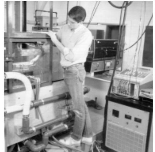
Jet impingement studies with application to the cooling of primary metals processing. Heater and temperature measurement module are developed for monitoring local heat transfer to an impinging liquid jet (1987).
